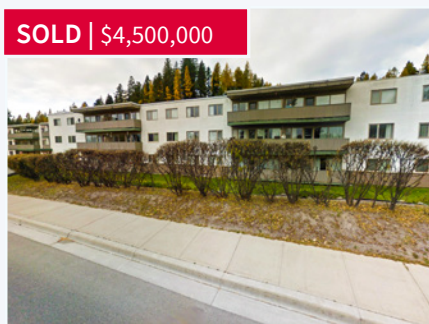
2655 Warren Avenue, Kimberley
